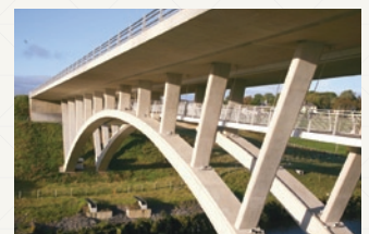
Irish Concrete Society – Design and Construction Award, winning entry in 2006 – 50% GGBS (insitu and precast concrete)
